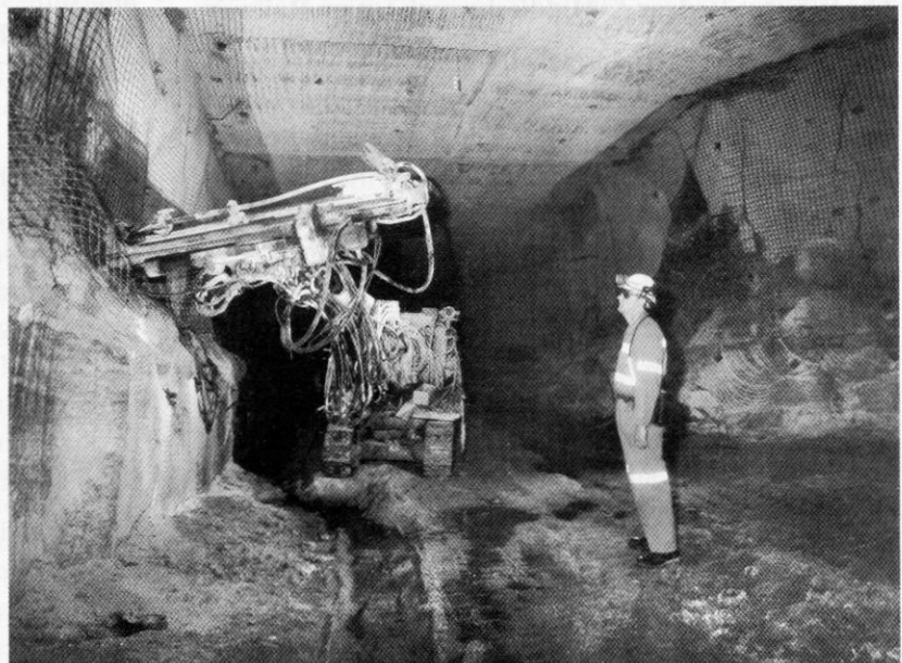
Rock bolting in progress – Photo by Paul Deakin
